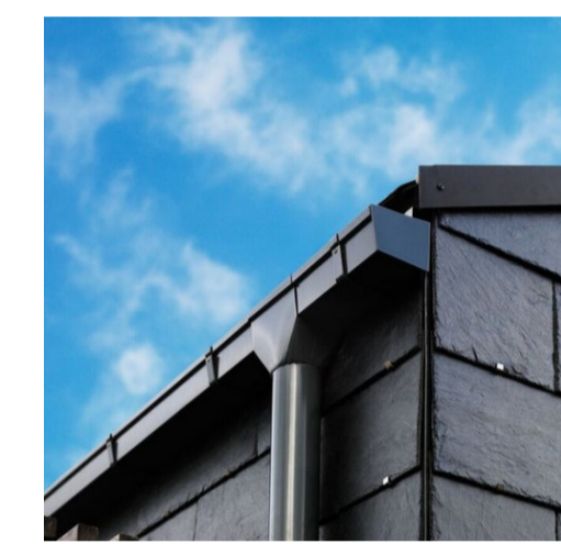
Aluminum box guttering
