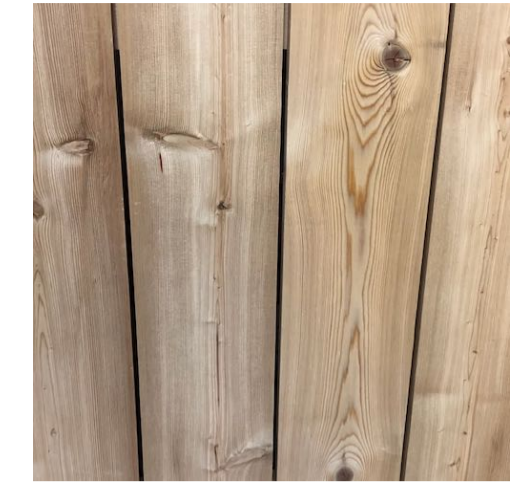
150mm vertical timber cladding boards
